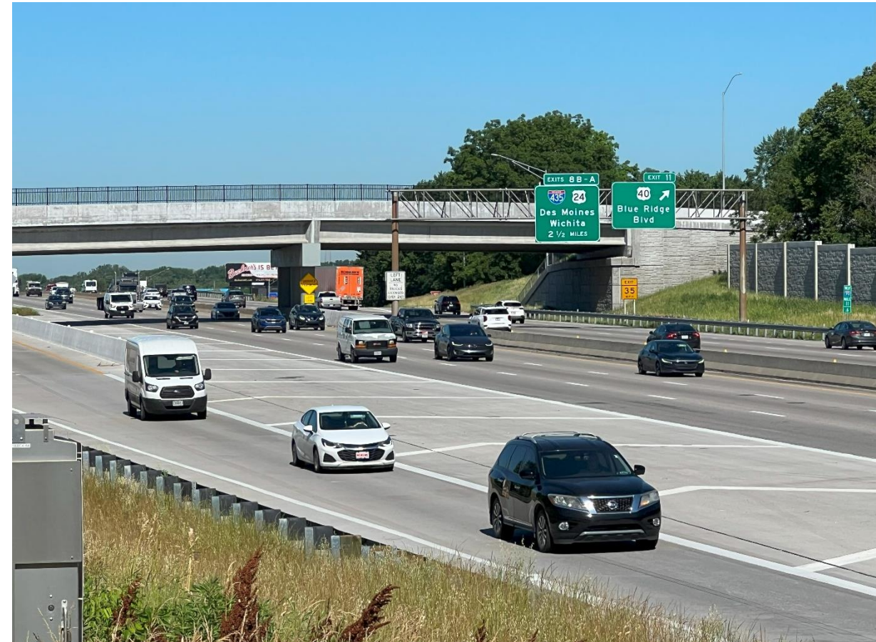
West view of I-70 on Blue Ridge Boulevard overpass
