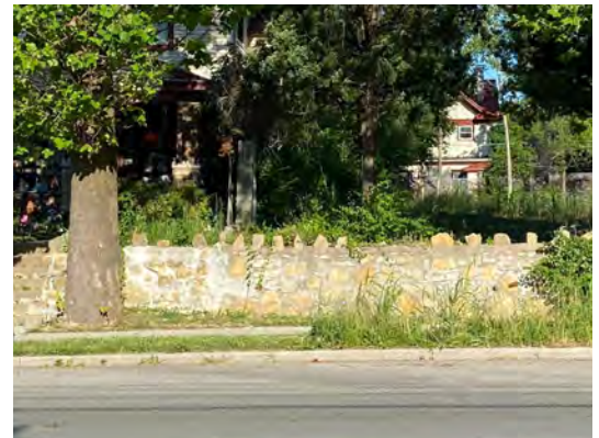
An existing stone residential retaining wall on Prospect.
