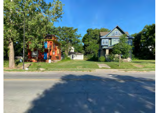
Renovated neighborhood housing on Prospect north of 35th Street.
