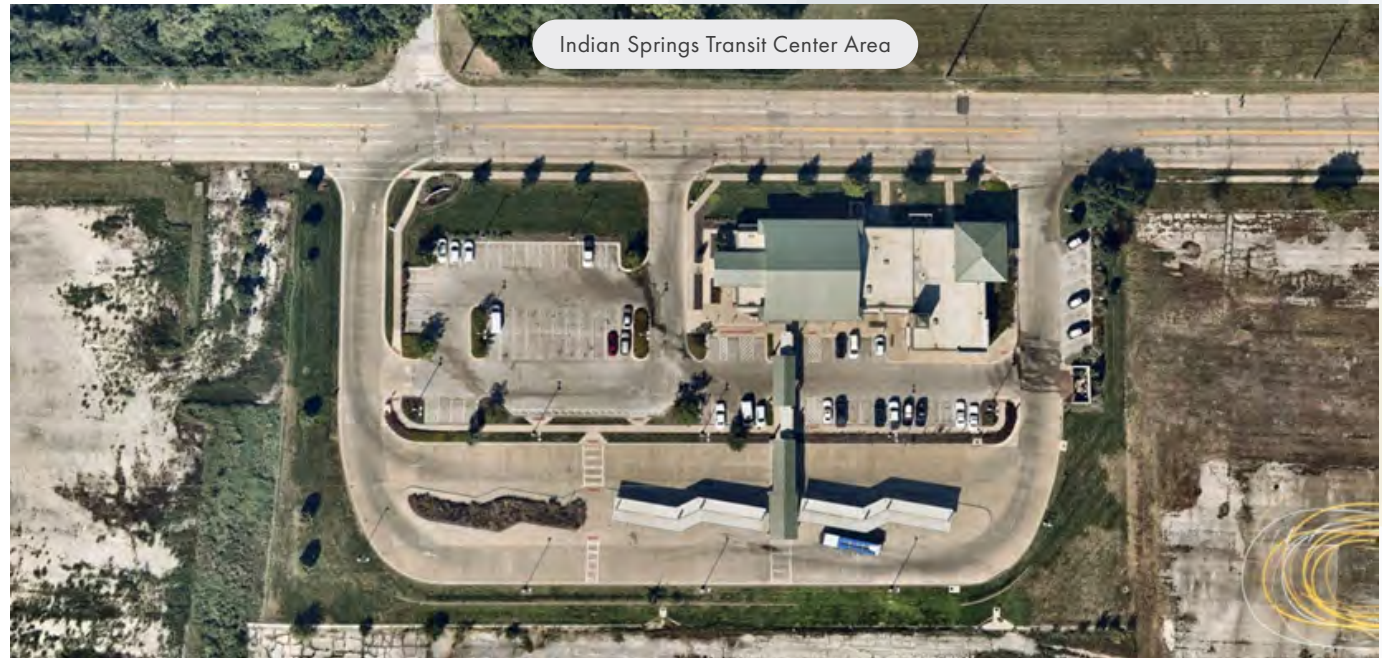
Figure 16. Potential Interim Pick-up / Drop-off Point at Indian Springs Transit Center in KCK
