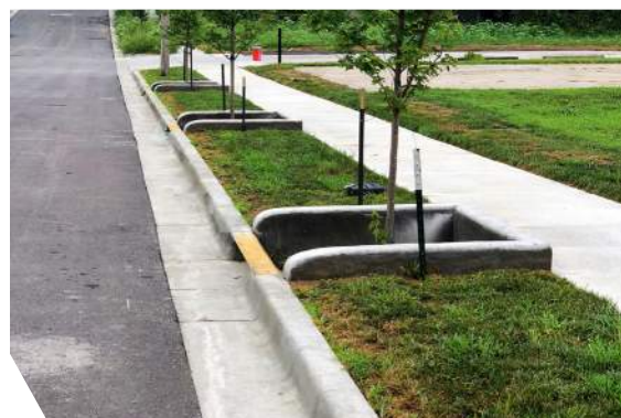
Roll Back Curb and Gutter
