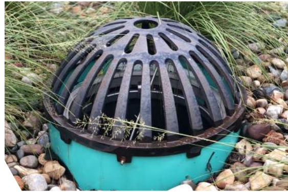
Manufactured Overflow Riser
