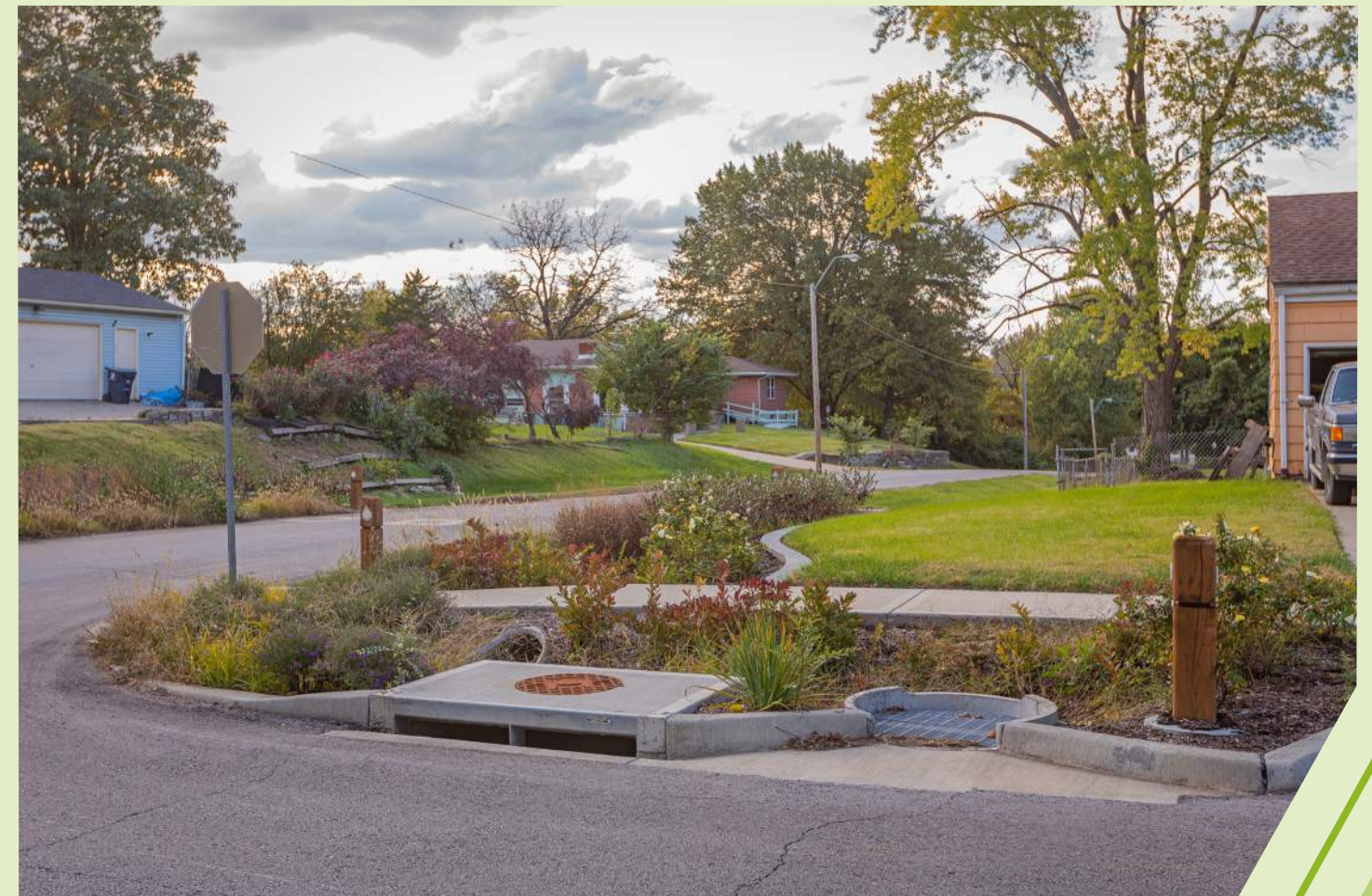
Inlets at 74th Street Rain Gardens
