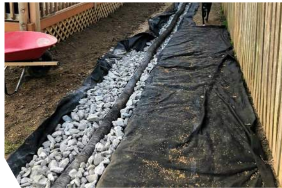
HDPE Underdrain Pipe
