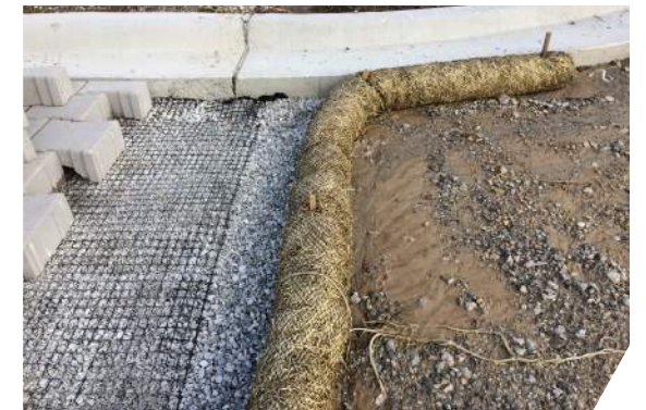
Surface Protection Before Rain
