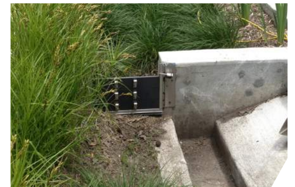
Manufactured Surface Weir
