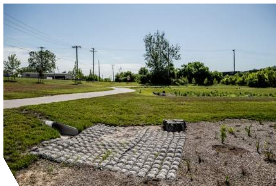
Tied Concrete Block Mat
