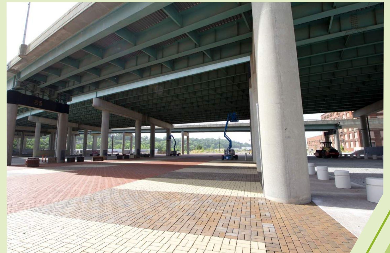
Permeable Pavement beneath I-670 Underpass in West Bottoms
