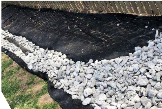
Permeable Geogrid Liner
