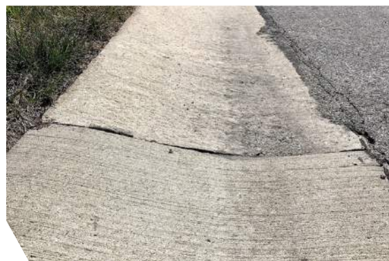
Reverse Roll Back Curb and Gutter
