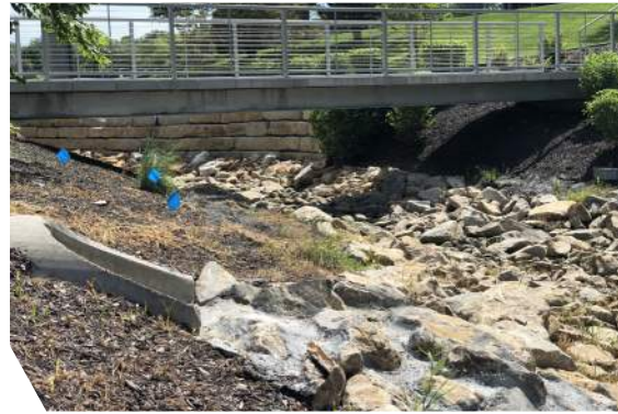
Concrete Embedded Splash Pad
