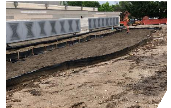
Erosion Control Log
