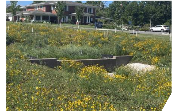
Stacked Stone Surface Weir
