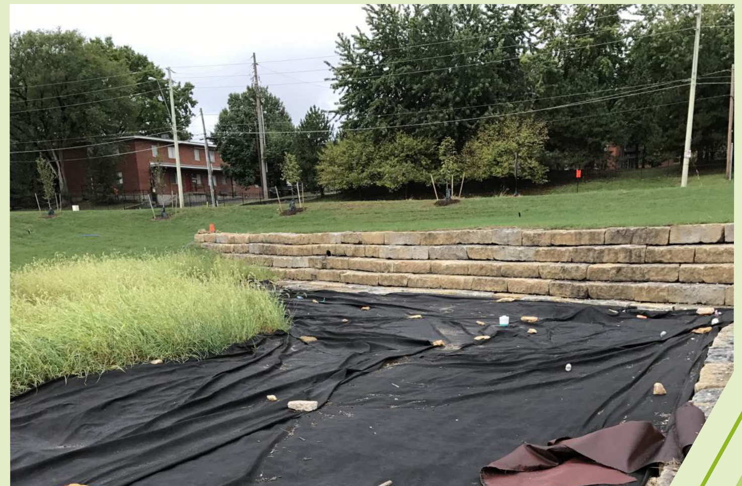
Liner Installation at 81st & Troost
