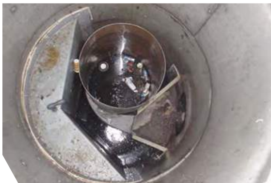
Catch Basin Insert (MARC BMP Manual, 2012)
