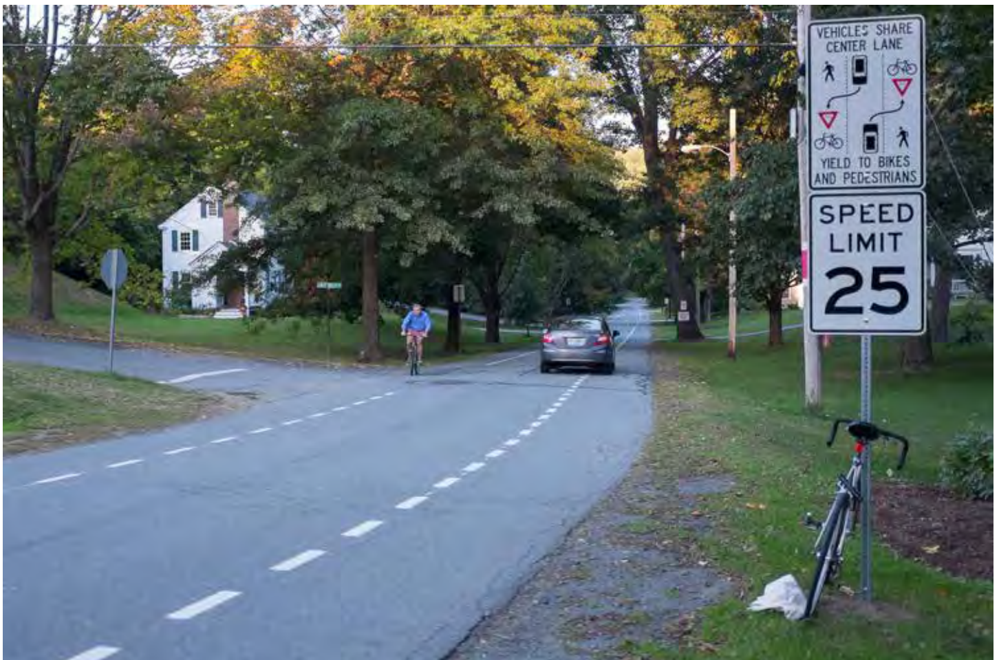
Advisory bike lanes are an option for constrained roads with low traffic.
