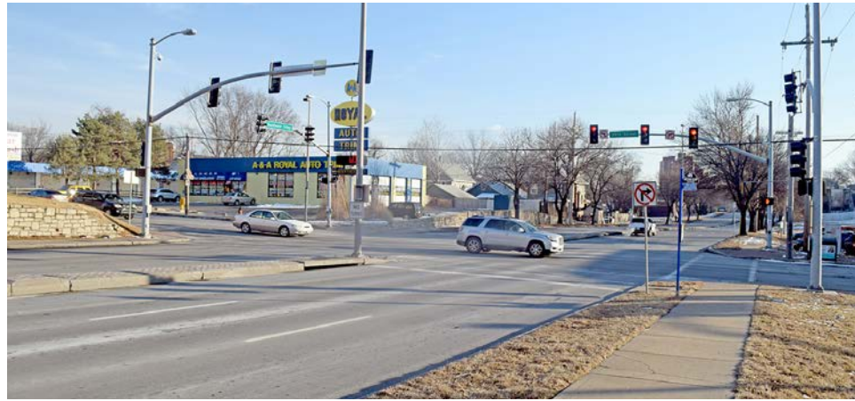
Bad Transit Facilities
