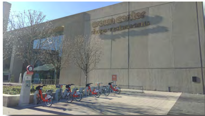
Crown Center Shopping Center
