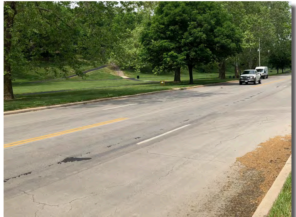
Gillham Road south of 44th Street looking North
