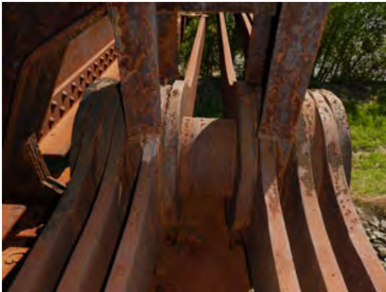
typical pinned connection of main span
