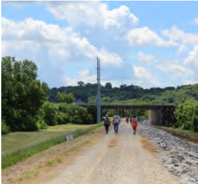
levee trail on top of embankment
