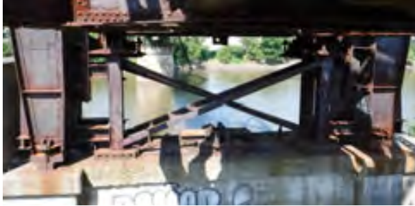
permanent blocking at supports
