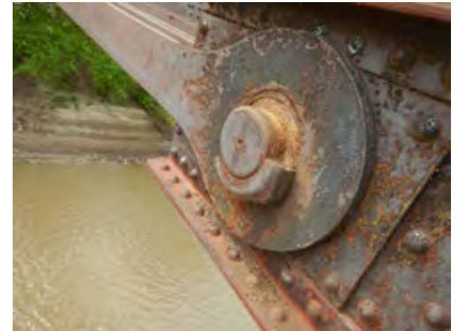
broken Lomas nut at pin
