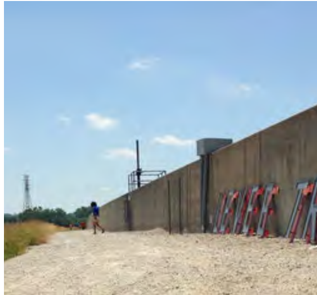
levee trail on inside of levee wall
