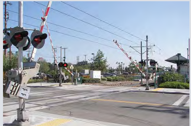
Fig. 3.23 – Example of a quad gate installation that would reduce noise and improve vehicular and pedestrian safety.
