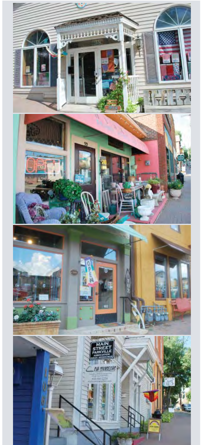
Fig. 3.46, 3.47, 3.48 & 3.49 – The existing storefronts along Main Street represent a broad range of materials, styles and finishes.
