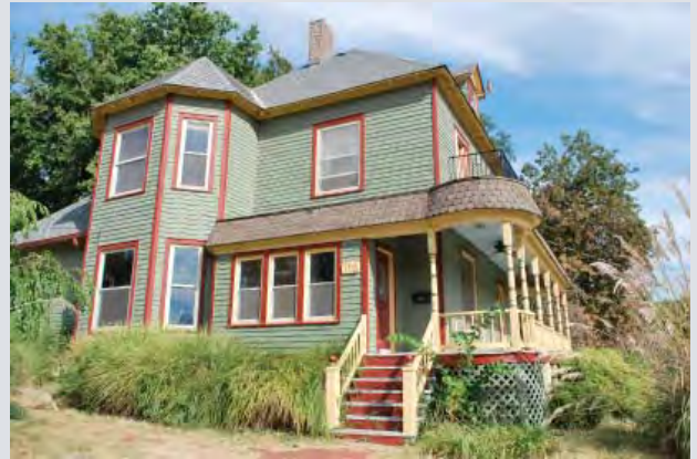
Fig. 3.1 – Example of the historic character to be preserved in the residential neighborhoods.
